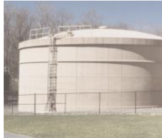
0.6 MG TES tank at the UPS data processing center in Mahwah, NJ
