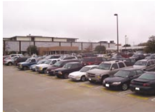
5.2 MG TES tank buried beneath the parking lot of an electronics manufacturer in Dallas, TX
